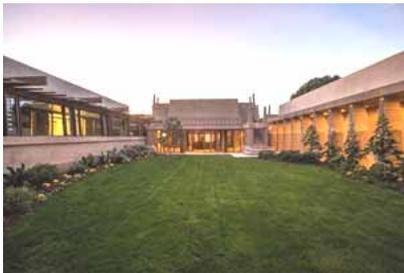
The architectural design features exterior walls that are tilted back at 85 degrees (which helps provide a "Mayan" appearance sometimes referred to as the Mayan Revival style, leaded art glass in the windows, a grand fireplace with a large abstract bas-relief, and a moat. Water is meant to flow from a pool in the courtyard through an underground tunnel to this inside moat, and out again to a fountain.
